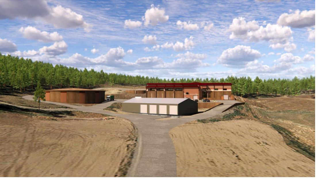
One option is to build the new WTP into the side of a sandstone bench, which would require only a single level of visible construction at the top. We are currently evaluating whether a drinking water storage tank is necessary for the WTP.
