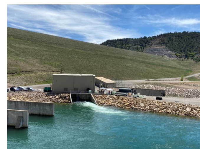
Pilot Site at Ridgway Reservoir Dam
